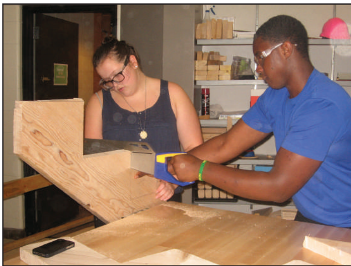
Students Tally Dully (lt.) and Alex Hilliard team up to build a stair stringer for the "Geometry in Construction" house.
