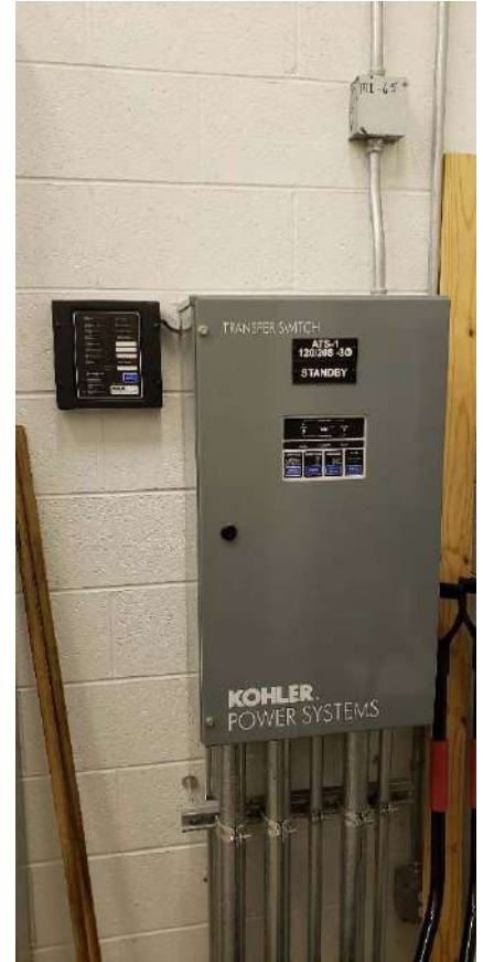
Photo #3 AT-1 and Remote Annunciator
