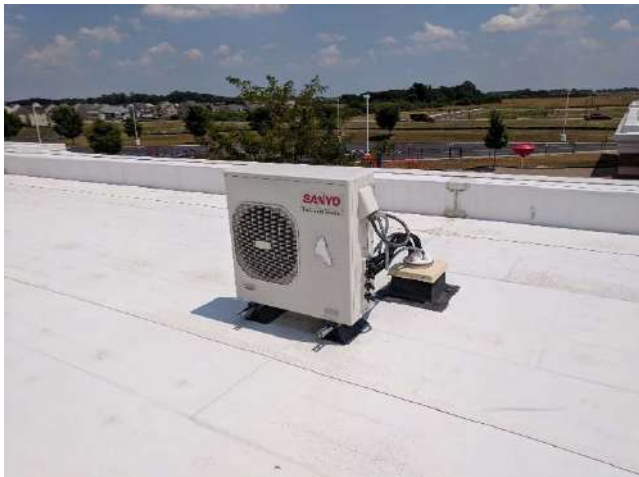
Photo #11 Typical Split DX Condensing Unit
