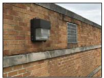
weathering of mortar joints has occurred, particularly around stone copings and windowsills. Walls show evidence of chronic wetness around downspout and overflow locations. A program of masonry cleaning and repointing in the mid-term future will help preserve strength and appearance.
