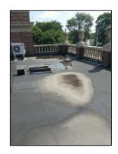
membrane, require attention. In particular, vertical membrane flashings were installed to cover and protect weathered brick parapets. Many of these are beginning to un-adhere and delaminate from the substrate. These should be repaired or reinstalled with additional fastenings and termination bars.
