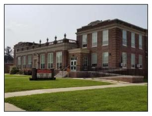
original roofs in low-slope areas have been replaced with EPDM membrane roofing systems, some in 2014 and some prior. However, some roofing issues require attention, particularly in the older replacements. The Auditorium roof is a sloped structure and is shingled; shingles show sign of weathering. The Gymnasium has a barrel vaulted roof with an adhered EPDM membrane roofing system.
