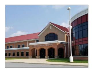
Similar to the adjacent Middle School, the exterior envelope is brick and split-face masonry in varying colors, with some areas of ribbed metal wall panels at upper areas. Masonry is in fundamentally good condition throughout. Large aluminum storefront / curtainwall, windows, and exterior doors are in generally good condition throughout, and include insulated glazing.
