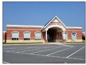
condition, but shows cracking and deterioration. Aluminum storefront, windows, and exterior doors are in generally good condition throughout, and include insulated glazing.
