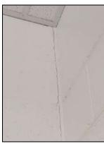
including corridors, toilet rooms, core amenities, and inside face of exterior walls are painted masonry. Interior walls are in good to fair condition. Select areas should be repainted, including incidental patching as required. Masonry walls and partitions show significant cracking in localized areas, which requires repair and repainting. This work is outside the scope of typical incidental touch-up by district personnel.
