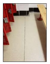
life, and should be replaced with new carpet and resilient base trim. Core area terrazzo floors are in good condition, with localized cracking that requires correction.
