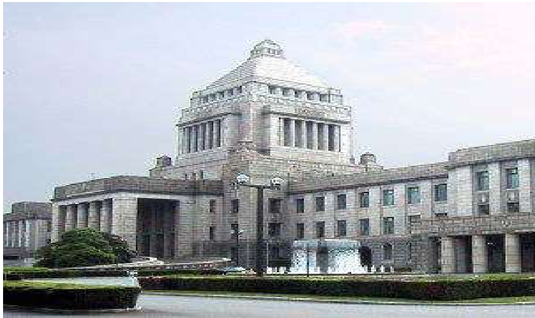
Above: Japanese National Diet Building
