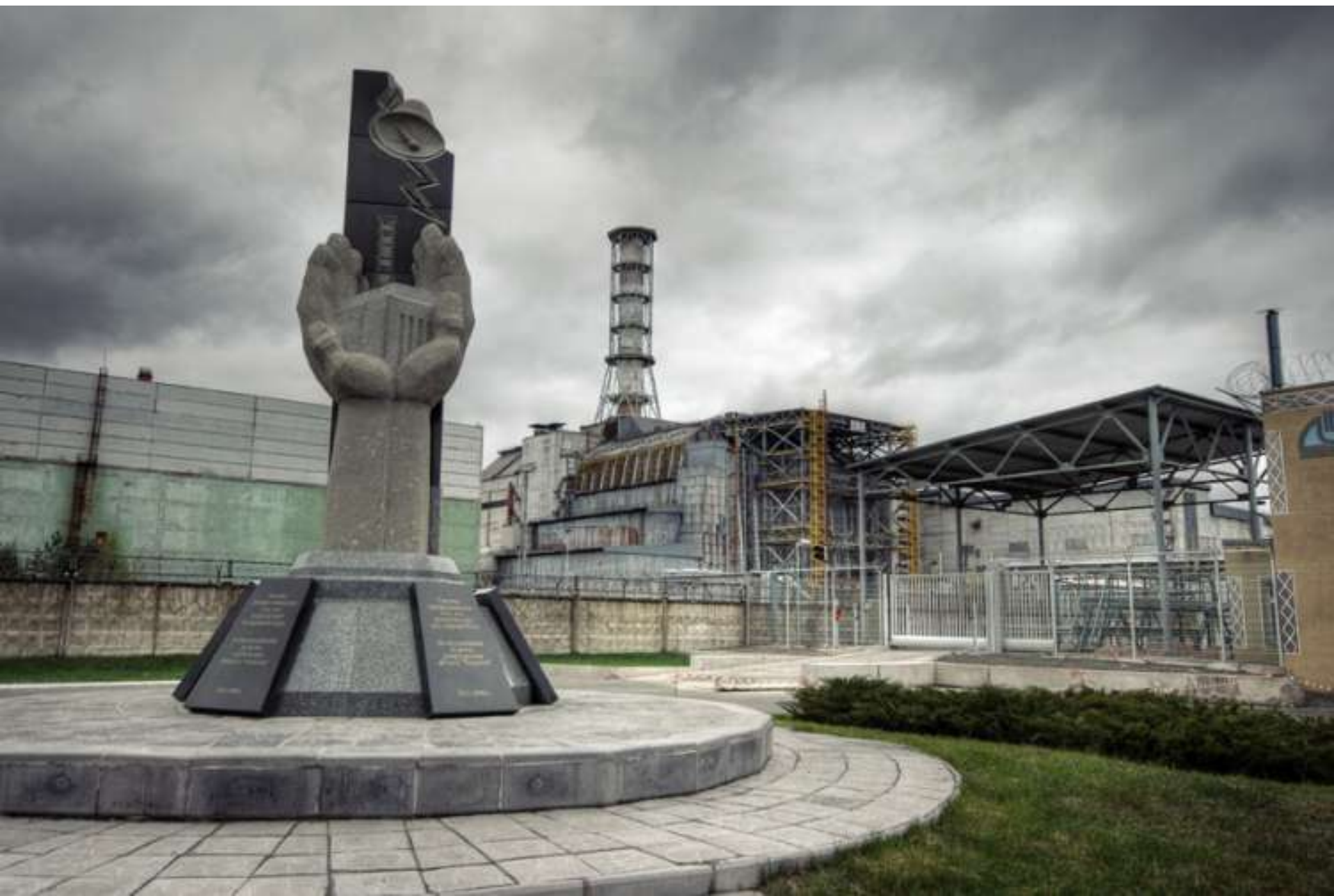
This monument is a remembrance of the people who died sealing the radiation leak.
