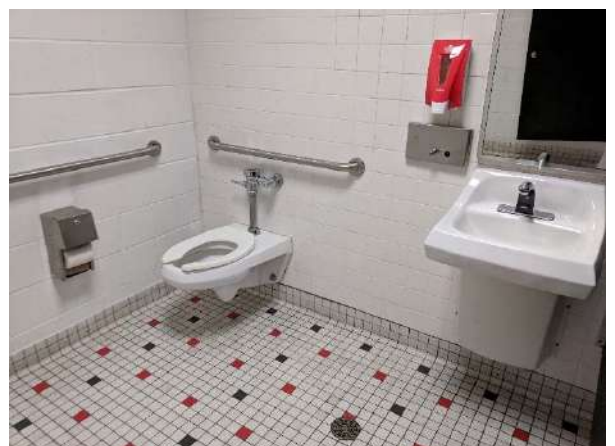
Photo #10 Typical Bathroom Lavatory
