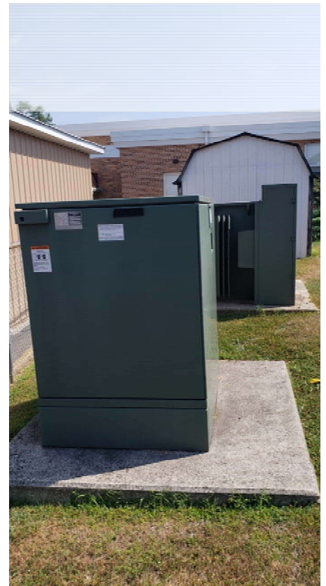
PMH-3 Switch and 500kVA Transformer
