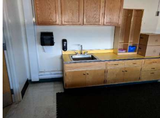
Photo #16 Typical Classroom Sink
