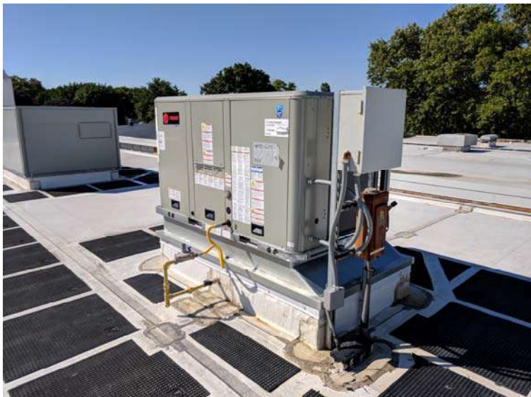
AHU-2 Rusty Disconnect Switch
