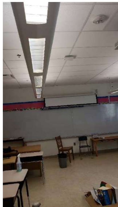
Photo #9 Typical 2006 Addition Classroom
