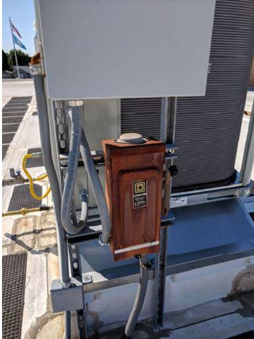
AHU-2 Rusty Disconnect Switch (B)
