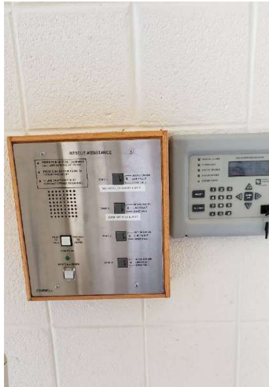
Photo #6 Rescue Assist Station and Fire Alarm Remote Annunciator
