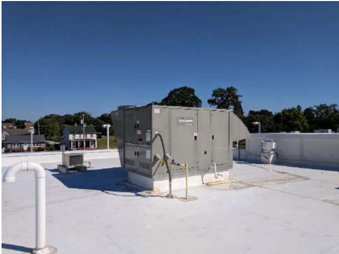
Packaged DX Rooftop Air Handling Unit serving Kitchen
