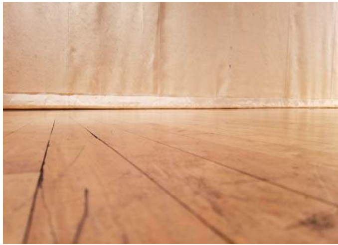
UNSEATED FIRE CURTAIN
