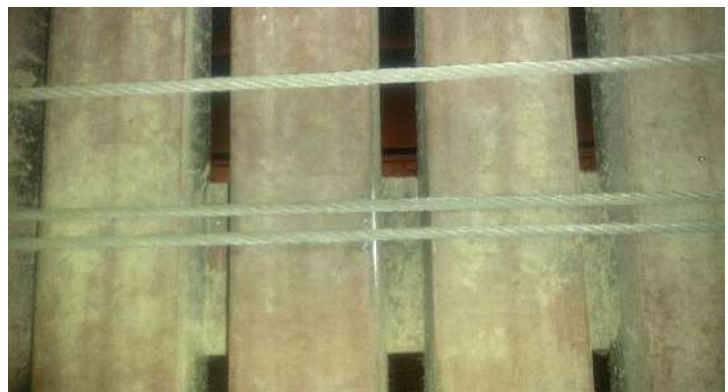
CABLES RUBBING GRID
