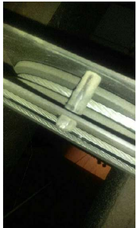
SHAVED KEEPER PINS: LOFT BLOCK
