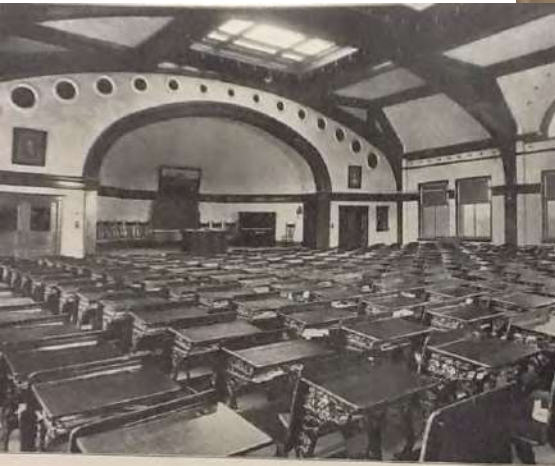
ASSEMBLY ROOM - FRONT VIEW
