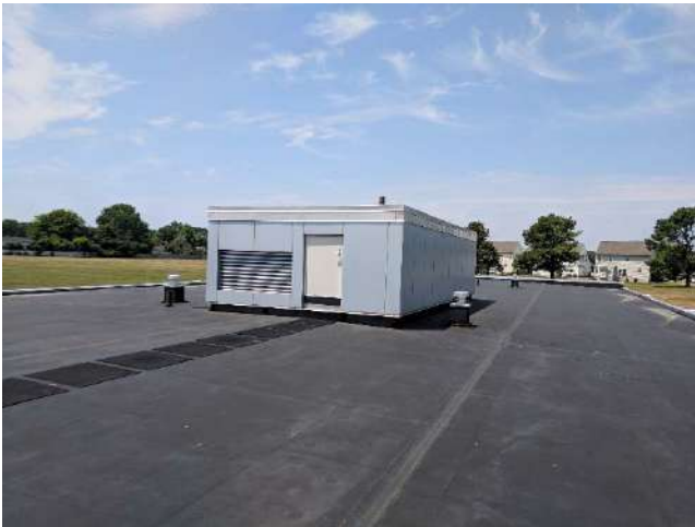
Photo #7 Mechanical Penthouse on Roof
