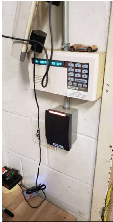
Photo #7 Security Keypad and Card Reader
