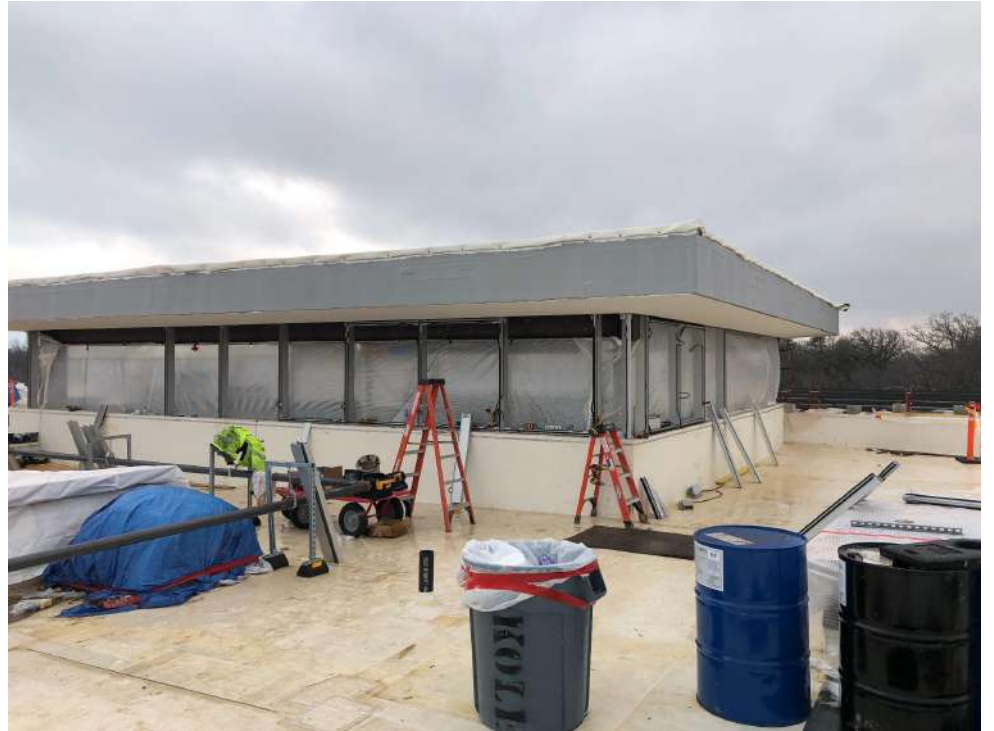
Clerestory Installation at South Vestibule/Tower
