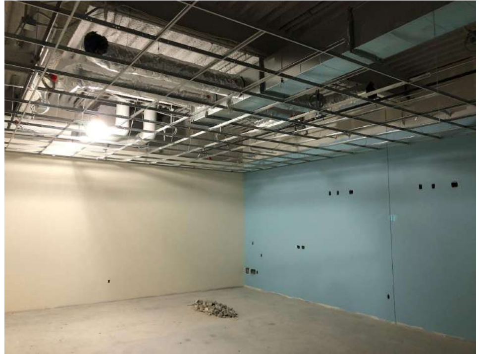
Painting and Ceiling Grid Install
