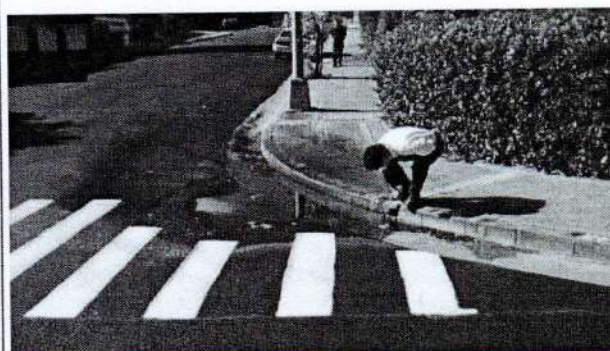
Curb drains typically convey runoff directly to the City's street drainage system without the benefit of absorption by permeable surfaces and natural treatments such as landscaped areas and planters.
