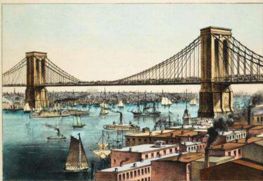
THE GREAT EAST RIVER BRIDGE.
