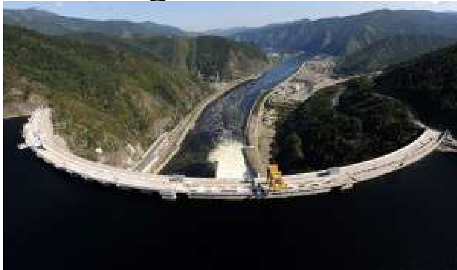
Above: Sayano-Shushenskaya dam
