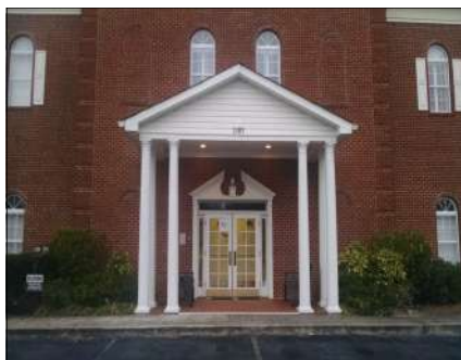
The Cumming VR office is located on Hwy. 9 across from Andean Chevrolet at the rear of the building.
