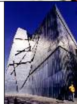
Jewish Museum Berlin Berlin, Germany This angular building is covered in thin sheets of zinc-titanium alloy. The untreated alloy will slowly oxidize and change color from exposure to the air and weather.
