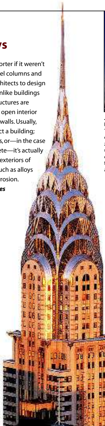
Chrysler Building New York City Completed in 1930, this steel-frame high-rise stands 319 m tall and features a distinctive spire sheathed in shiny stainless steel.
