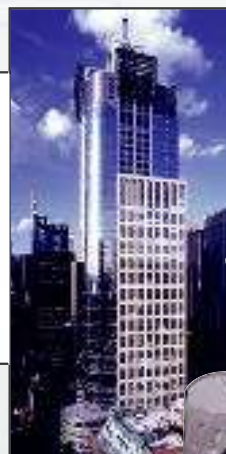
Condé Nast Building New York City 866 ft (264 m) tall, 48 floors
