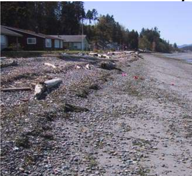
Shoreline seawall near Anacortes, WA.
