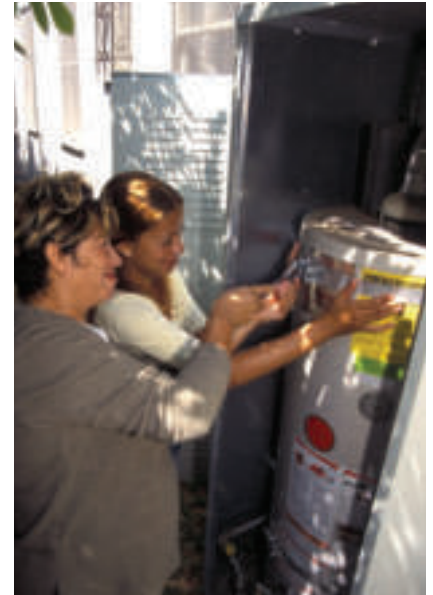
Figure 22 Sturdy metal straps on this gas water heater help reduce the danger of fires from broken gas lines during an earthquake.
