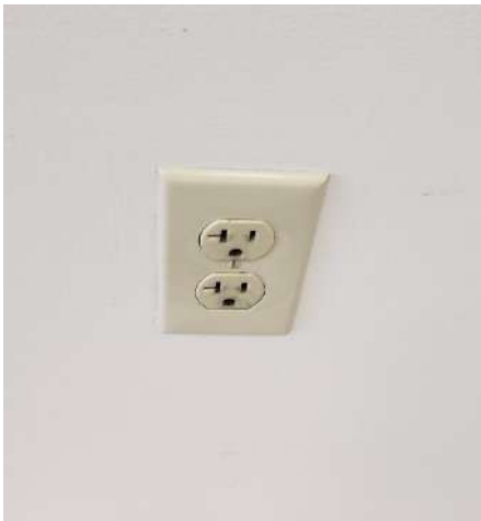
Photo #10 Typical Receptacle
