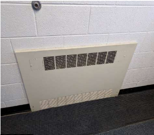
Photo #14 Typical Cabinet Unit Heater
