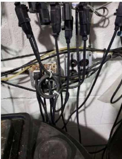
Photo #5 Receptacles in mechanical shop with evidence of rusting.
