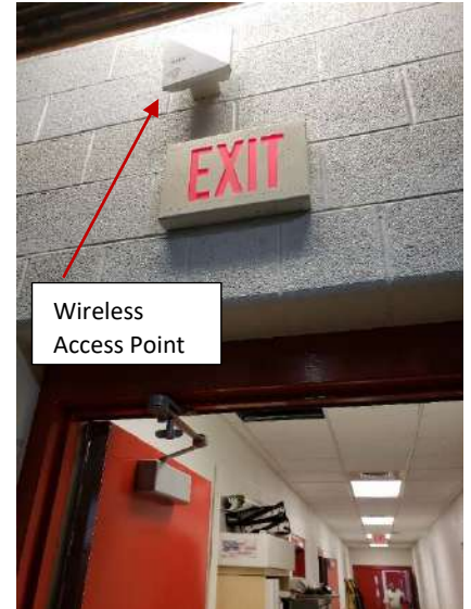
Photo #3 Typical Exit Sign and Wireless Access Point
