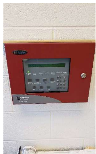
Photo #11 Remote Annunciator Panel
