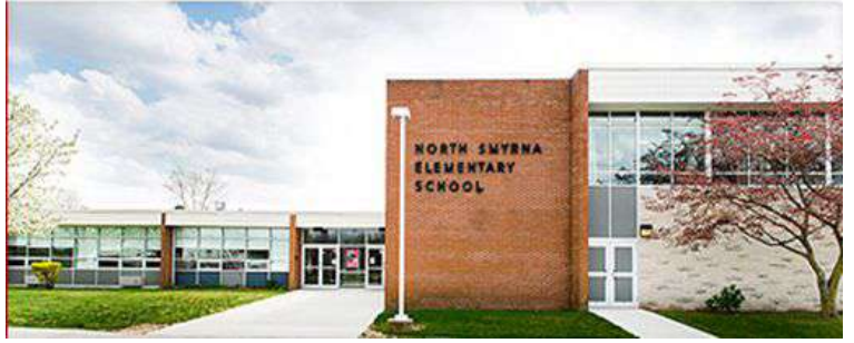
North Smyrna Elementary School
