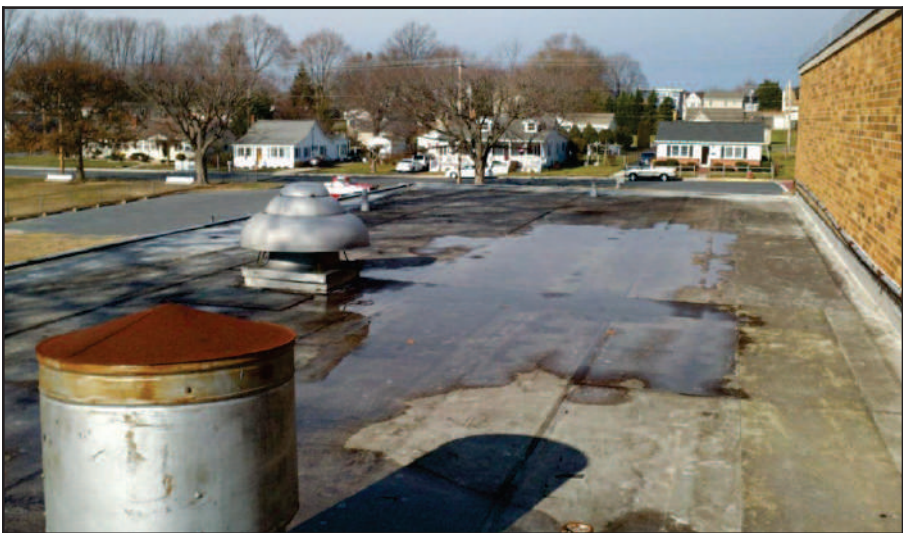
SES Roof - ponding & blistering due to exceeding lifespan
