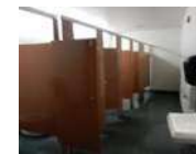
RESTROOM / ADA UPGRADES
