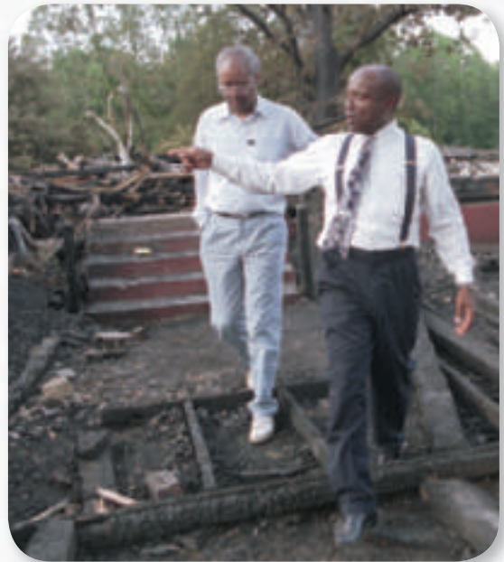
Surveying the damage
