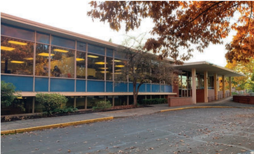
EXISTING VIEW – NORTHWEST
