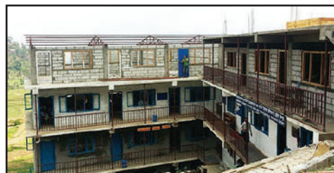
School under construction in Pharping, Nepal
