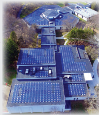
Beecher's blue roof? 970 solar panels now produce one-third of school's electricity - pg 11
