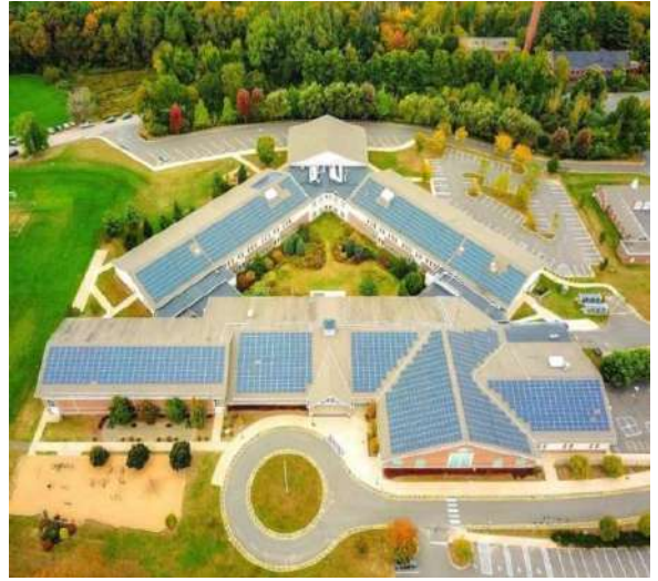
Reed Intermediate solar project completed 8/1/17 Size of system: 635,000 Watts
