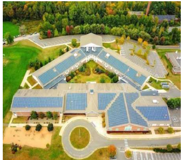
Reed Intermediate solar project completed 8/1/17 Size of system: 635,000 kW
