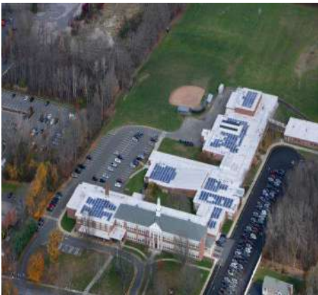
Newtown Middle School solar project completed in 5/1/13 Size of System: 180,000 kW
