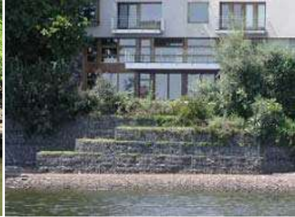
Figure 4: Gabion wall.
