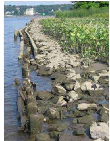
Figure 8: Degraded timber cribbing acts as a sill, protecting the tidal marsh to the shoreward.
