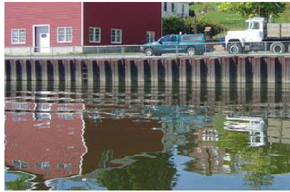
Figure 2: Steel sheetpile bulkhead.
