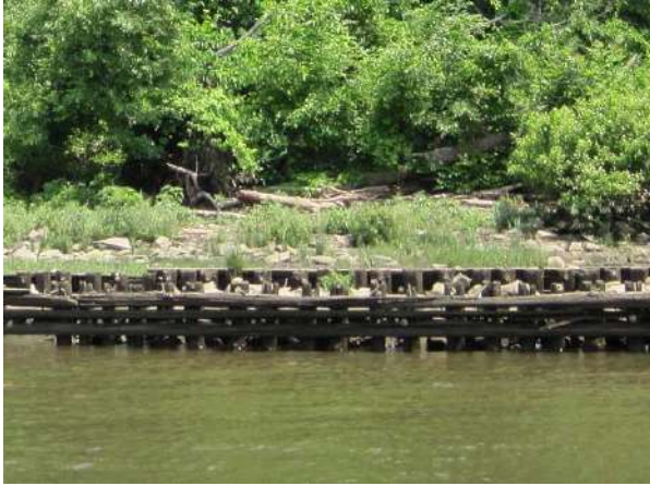
Figure 3: Degraded timber cribbing.
