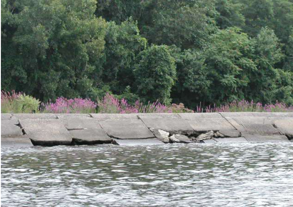
Figure 5: Failing concrete revetment.
