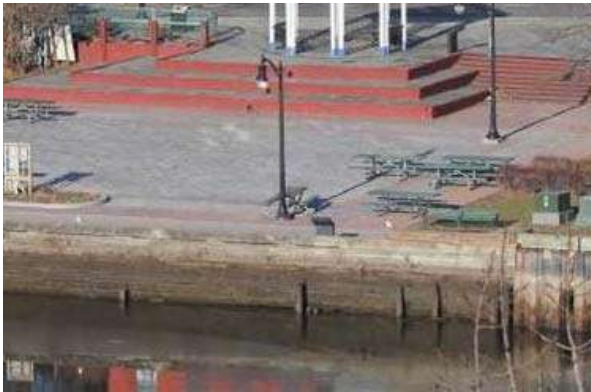
Figure 1: Timber bulkhead.
