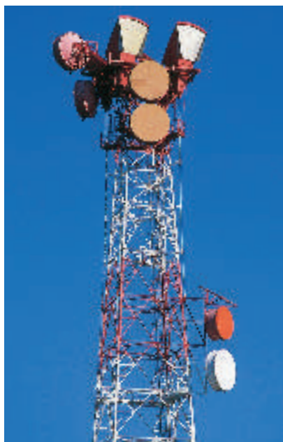
Figure 9 Towers such as the one shown here are used to send and receive microwaves.
