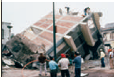
Figure 13 Effects of Subsidence Due to Liquefaction This tilted building rests on unconsolidated sediment that imitated quicksand during the 1985 earthquake in Mexico.
