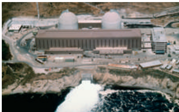
Figure 11 Diablo Canyon Nuclear Plant Near San Luis Obispo, California Reactors are in the dome-shaped buildings. You can see cooling water being released to the ocean.
