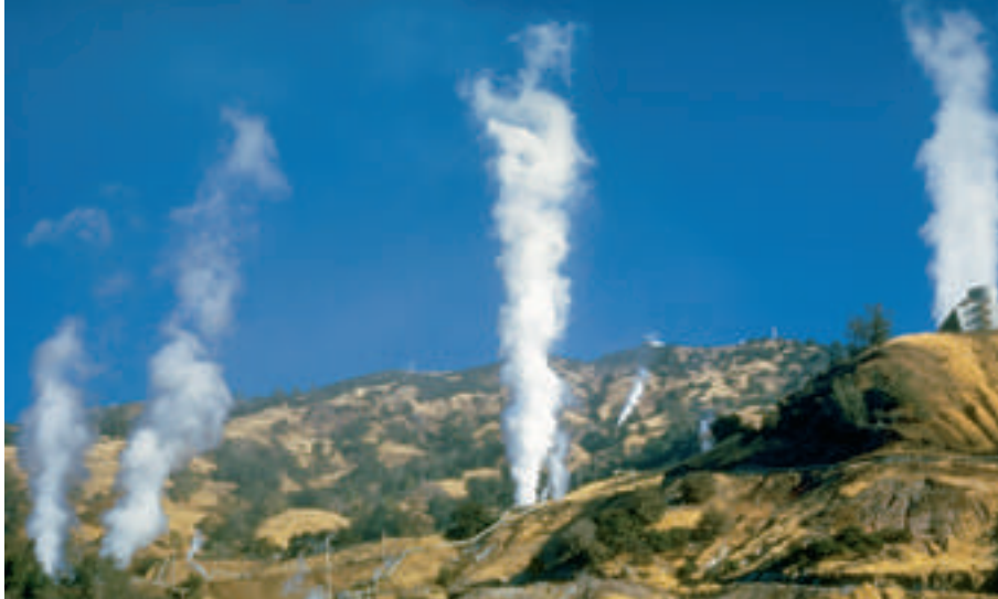
Figure 14 The Geysers is the world’s largest electricity-generating geothermal facility. Most of the steam wells are about 3,000 meters deep.
