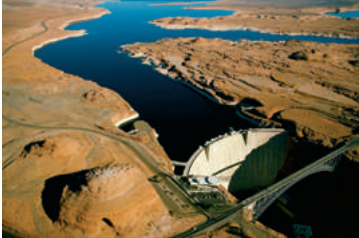
Figure 13 Glen Canyon Dam and Lake Powell on the Colorado River As dam operators release water in the reservoir, it passes through machinery that drives turbines and produces electricity.
