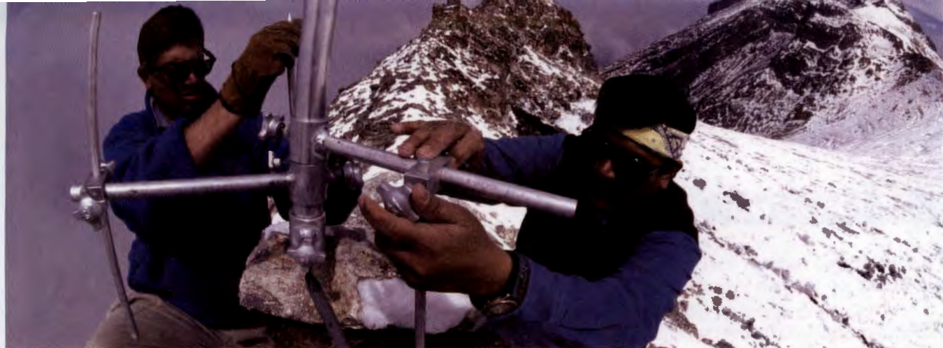
▲ Two engineers are installing communications equipment on a mountaintop.
