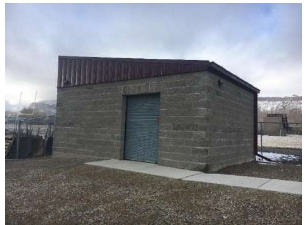
[The current storage building that will be converted for the project]
