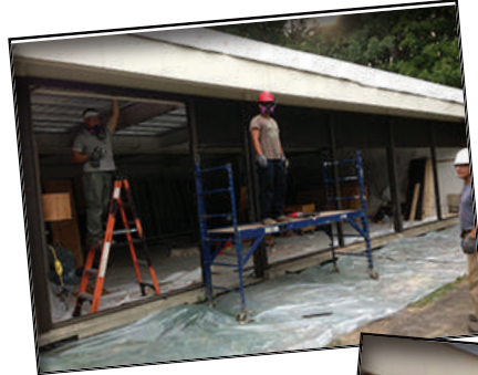
Tear down the old window wall.
