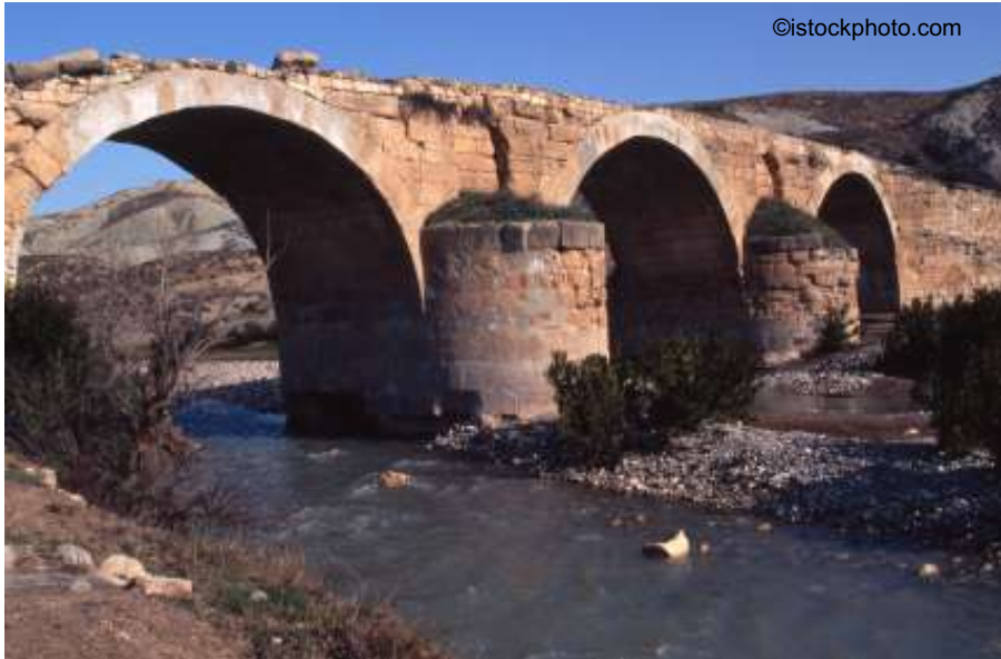
A Roman bridge crosses the Afrin River in northern Syria and is still in use today.
