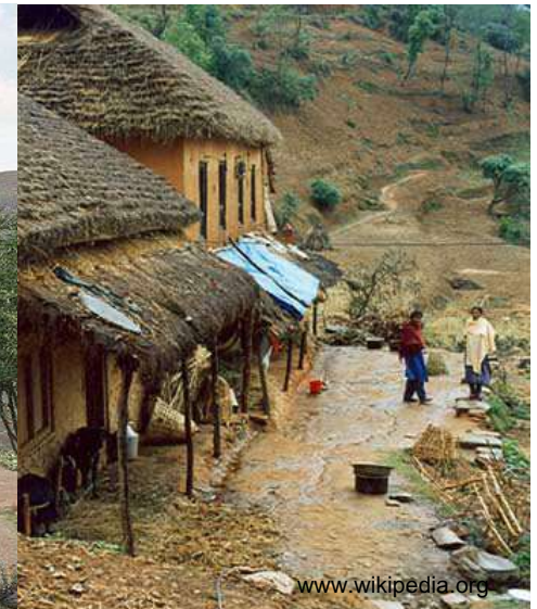
Nepalese house built of stone and clay
