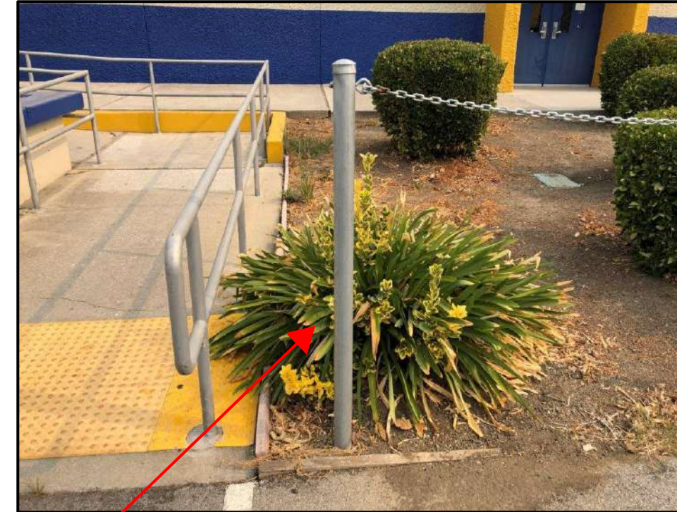
Photo 3: Trim shrub to accommodate for fence installation
