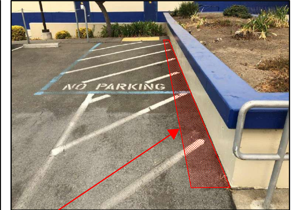
Photo 4: Black out with approved traffic marking paint from planter corner to end of asphalt paving 6" past top edge of seat wall. Do not paint over "NO PARKING" sign. Do not paint vertical planter wall.
