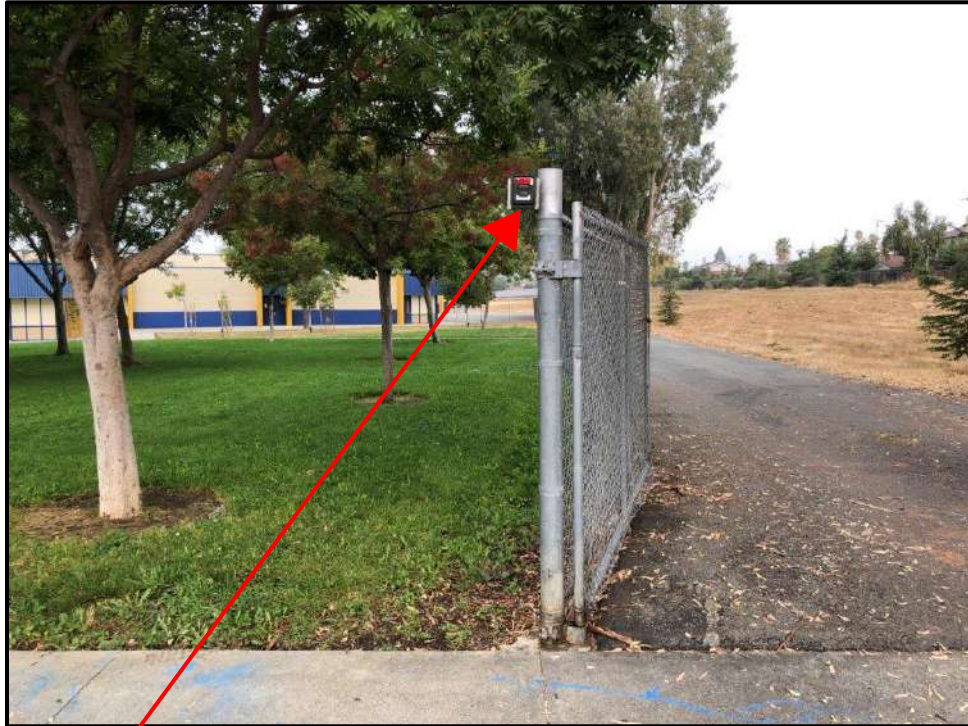
Photo 1: Temporarily remove knob box as necessary to accommodate for fence installation and reinstall at existing location.
