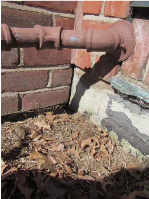
Opening in brick of exterior wall
