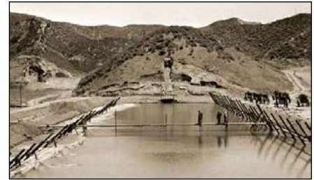
Dry Canyon Reservoir
