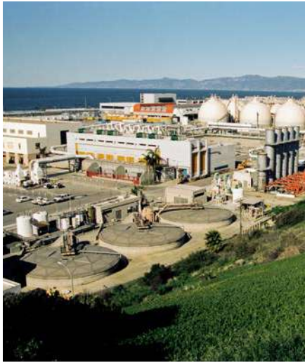
Hyperion Wastewater Treatment Plant, California
