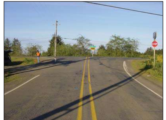
Westbound Drift Creek Road Approach
