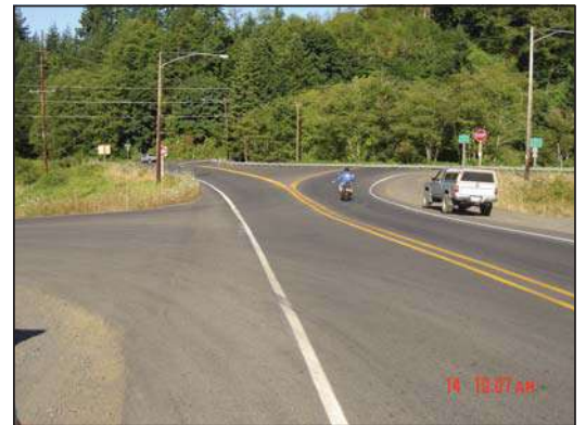
Northbound Business 20 Approach
