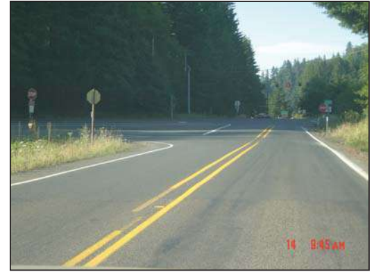
Southbound OR 229 Approach
