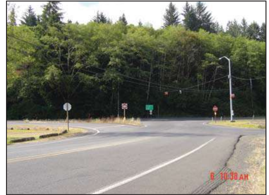
Southbound Old Scenic Highway Approach
