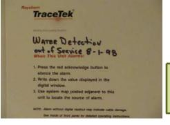
This water detection system has not functioned for a decade
