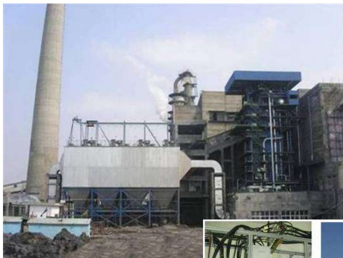
Left: Circulating fluidized bed
