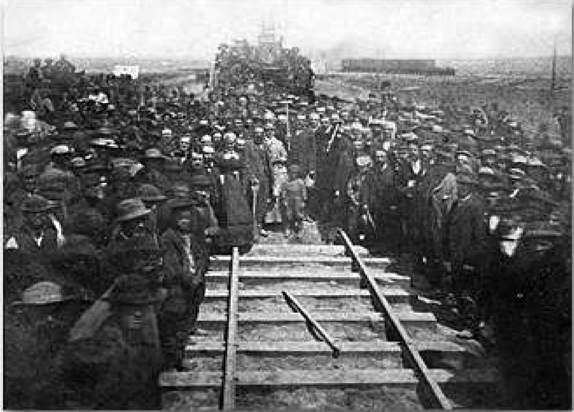
The Last Rail is Laid
