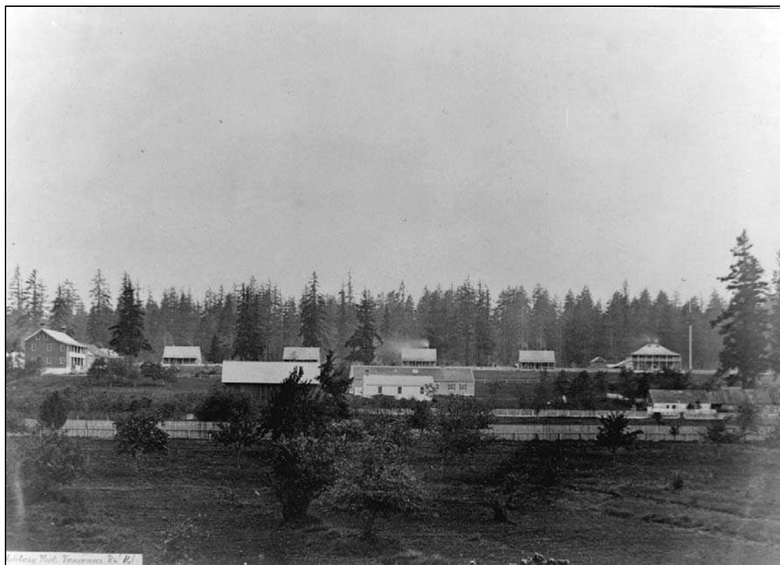
Figure 5. View of the northern edge of the HBC apple orchard as seen in the 1860 British American Joint Boundary Commission Survey image of the Vancouver Barracks Officers' Row. The Grant House stands in the right central portion of the image. (Image Courtesy of the National Archives of Canada).
