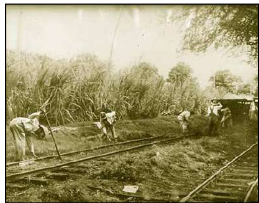
Filipino workers maintaining Pioneer Mill railroad line, n.d.
