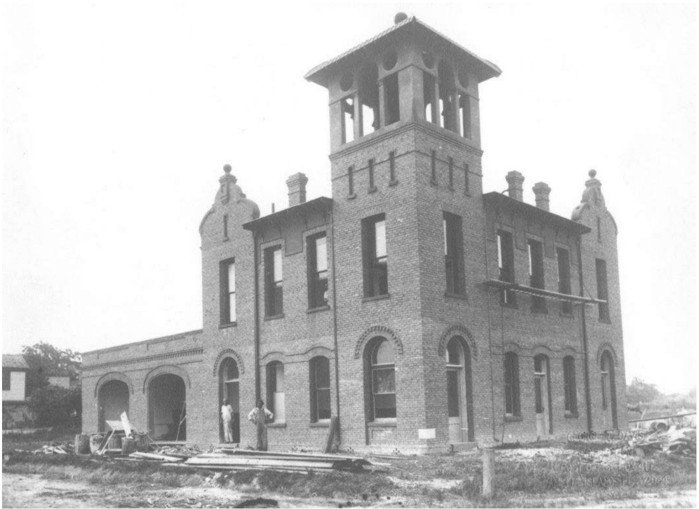
City Hall under construction. 1904
