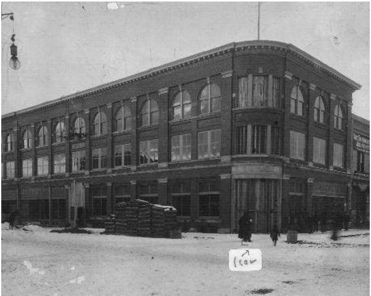
A recently found photo of the construction of this gorgeous building!
