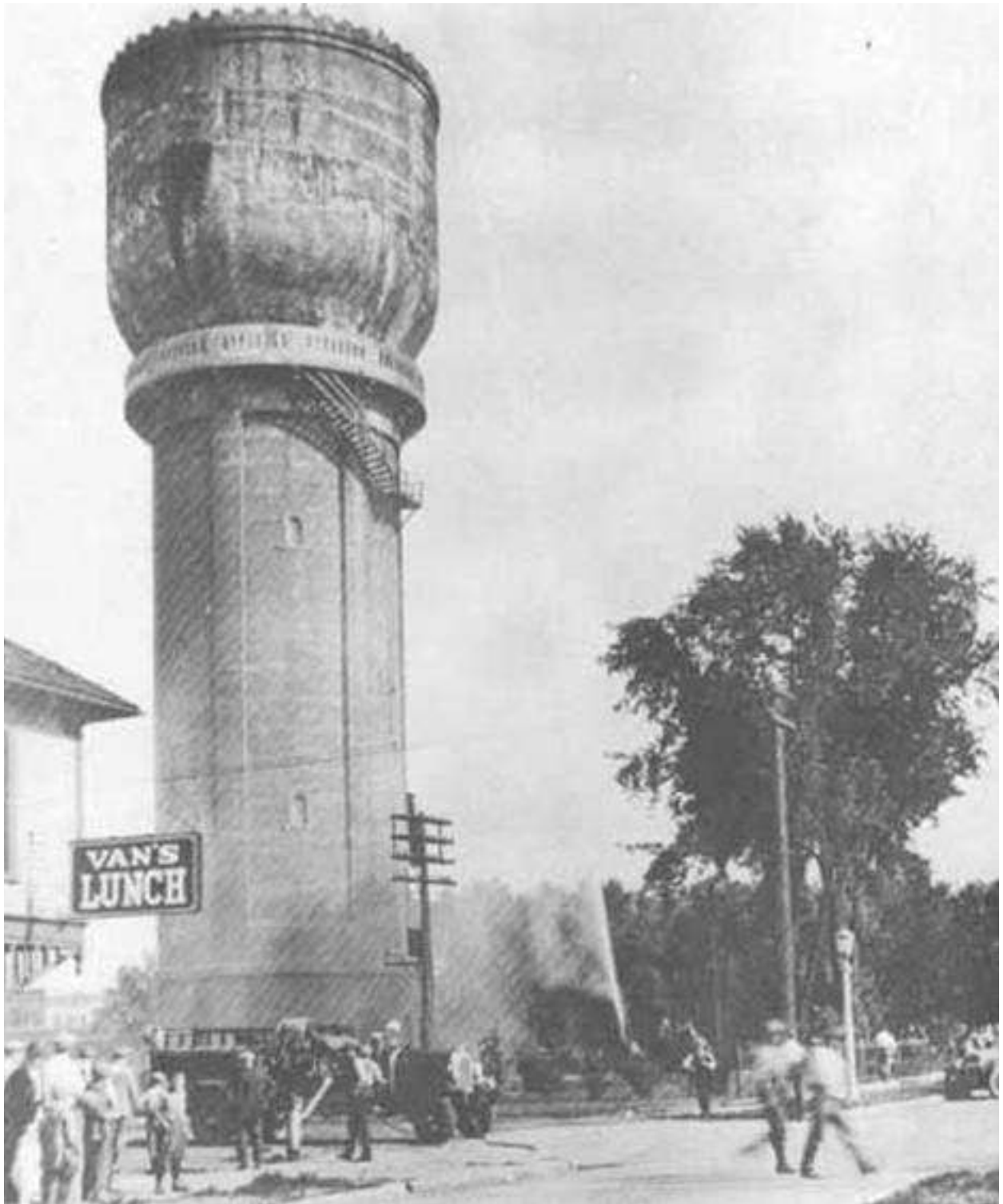
Testing New Fire Fighting Equipment c. 1927
