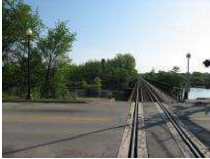
Railroad Bridge, today
