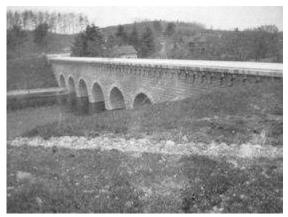
This hike ends near the aqueduct bridge over the Assabet River, a town landmark. The bridge was completed in 1897 to transport water across the Assabet River. An inverted siphon placed under the river in 1946 supplanted the leaky bridge crossing. Currently the aqueduct bridge is not accessible for walkers because of safety concerns. The picture shown here was taken around 1900 from the east side shortly after the aqueduct was built. Edmund Hill is in the background.
