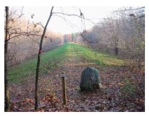
Earthen dams at two locations along this trail were designed and constructed by the U.S. Soil Conservation Service and state agencies for flood control after floods in 1955 damaged towns along the Assabet River. These dams were completed in 1963.
