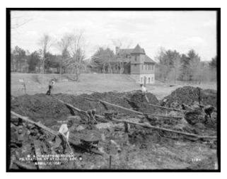
When this picture was taken in 1887 near the intersection of Bartlett St. and Lyman St., the Wesson pump house could be seen from the aqueduct then under construction. Water was pumped from Stirrup Brook by water power to an underground cistern near Wesson Terrace. From there the water flowed by gravity to the Wesson Estate (White Cliffs).
