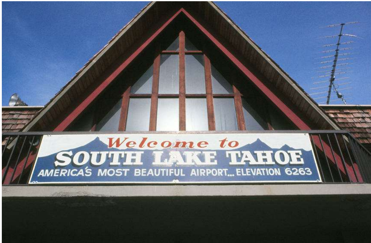
May 1975: One of the highest "airline" capable airports in the United States, Lake Tahoe's main passenger terminal building still holds that alpine charm as evidence from the A-framed construction and welcoming sign.
